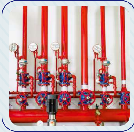
Fire Fighting and HVAC piping Installation
